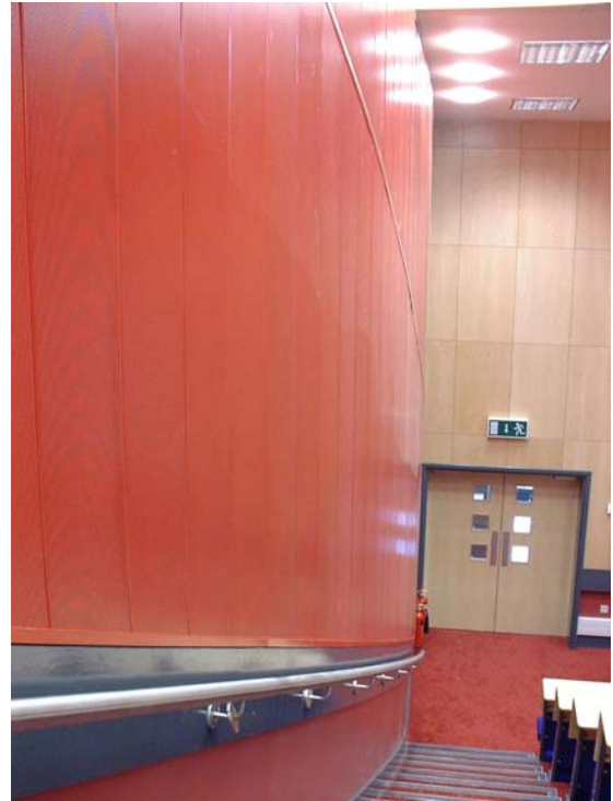
RC50MP Panels in lecture theatre
