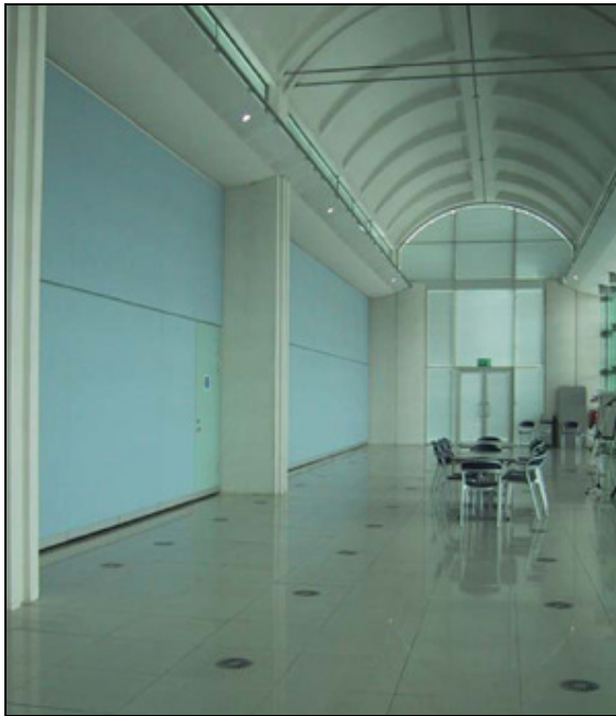
CP Wall Panels: Sheffield Millennium Gallery
