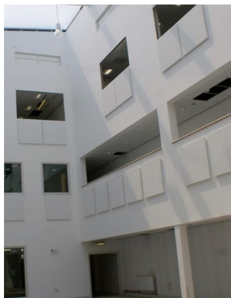
HA/W Squares mounted on atrium walls
