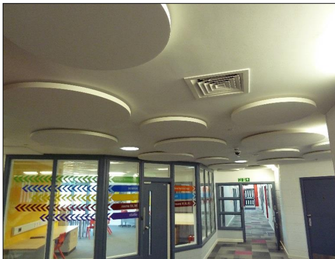
HA/W Baffles fitted to a ceiling (1200 dia disc)
